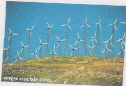
FIGURE 3.9 A Typical Wind Farm
