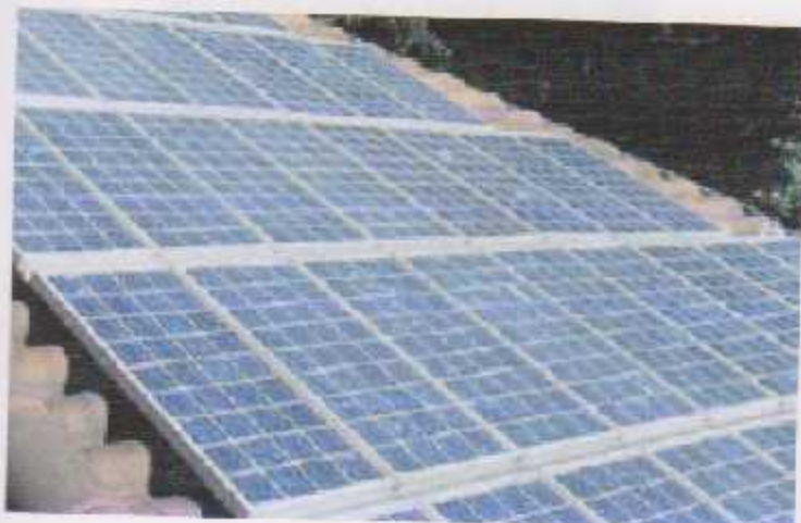
FIGURE 3.10 Discreetly blending in with roof tiles, solar panels
