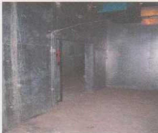
Figure (3-2) Photos Taken inside a Refrigeration Room
