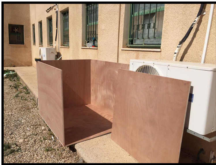
Fig (4.2) installation the container
