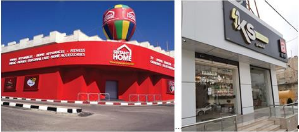
Figure 2.6: the use of Alucobond material as an external layer in Hebron commercial building
