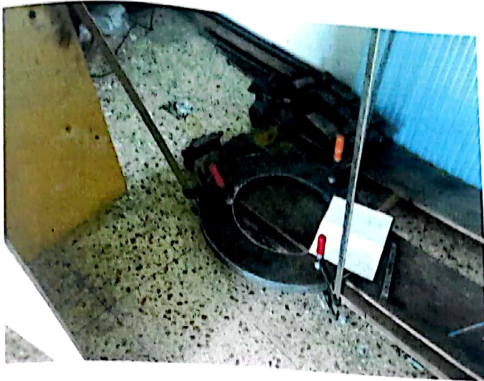
Figure (5.21): making the flanges fixed.
