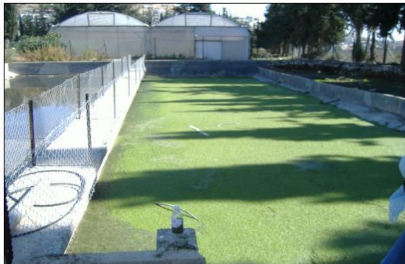
Figure 2.10: DW ponds system at Al-Aroub WW treatment plant adopted by Sharkh in 2007 [27].
