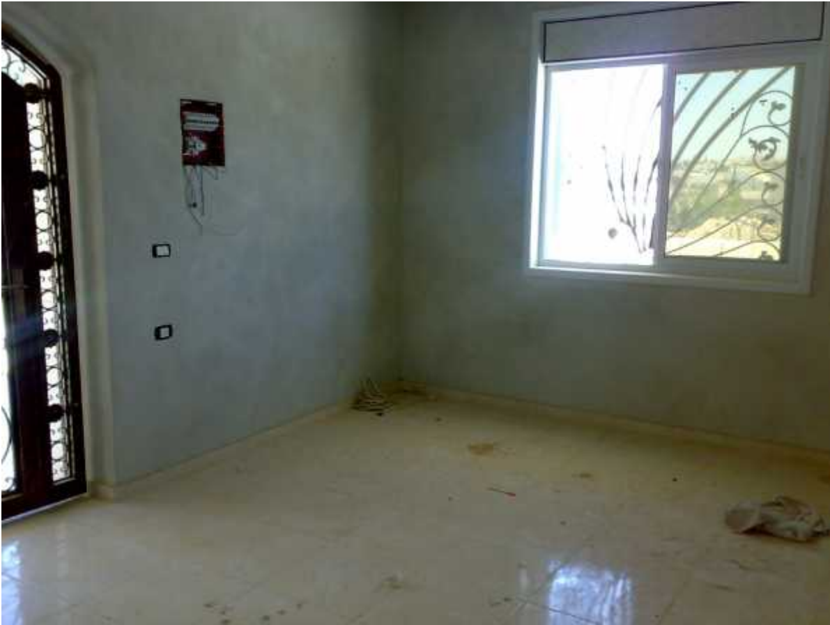
Figure 4.40: interior description of the tested room for class 8.
