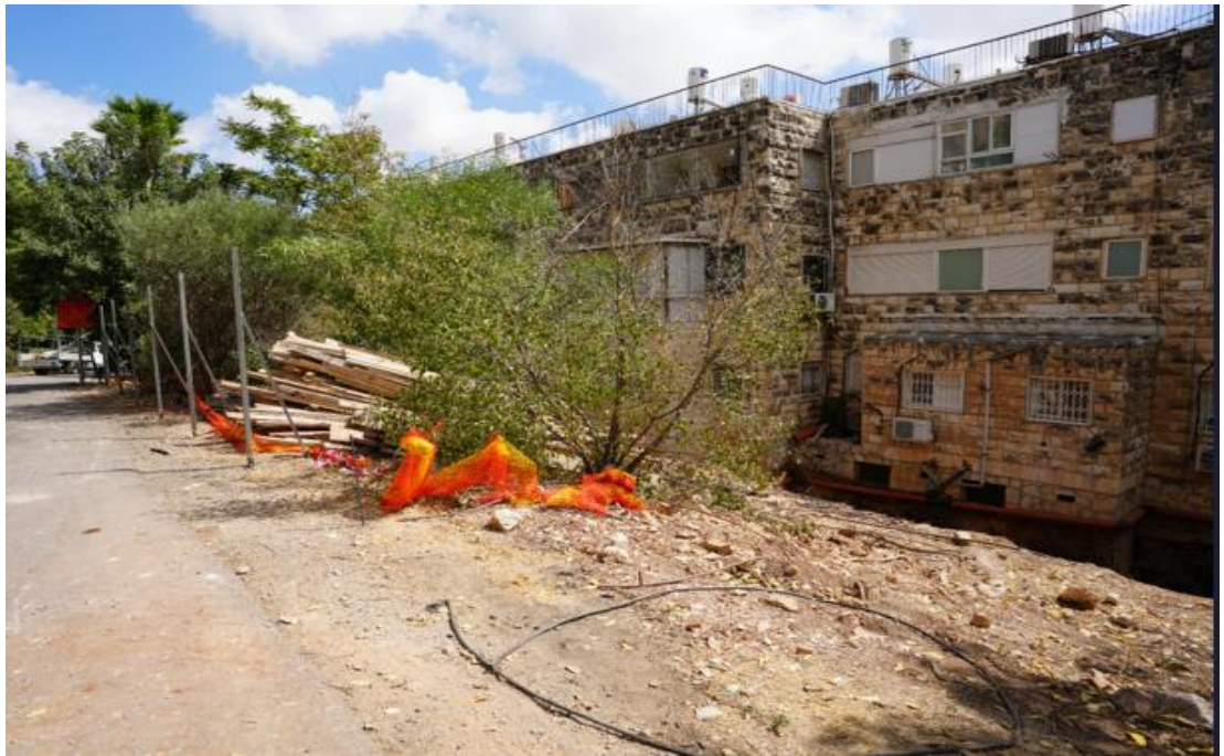
Figure 4.2 presents the general condition of the existing building prior to rehabilitation.
