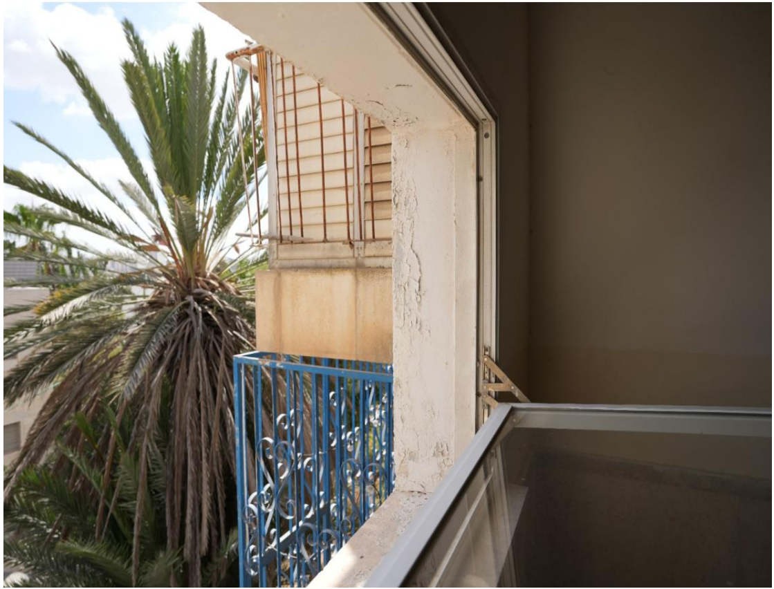
Figure 4.6: Representative condition of the existing structure showing adequate structural integrity despite localized age-related deterioration.
