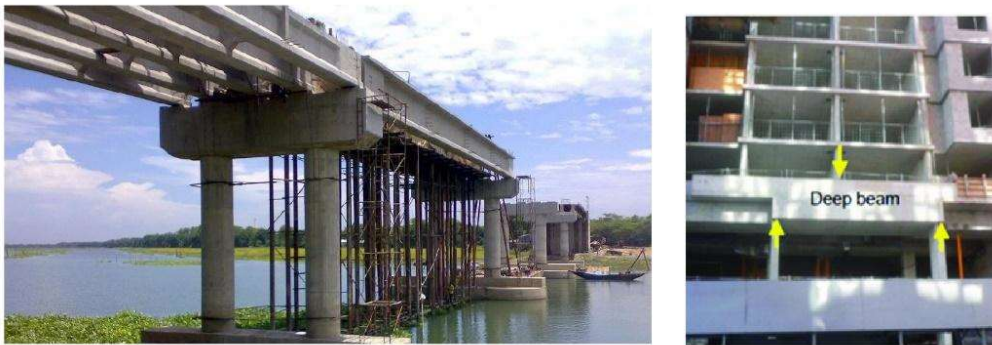
Figure 1. 1 Typical applications of reinforced concrete deep beams.
