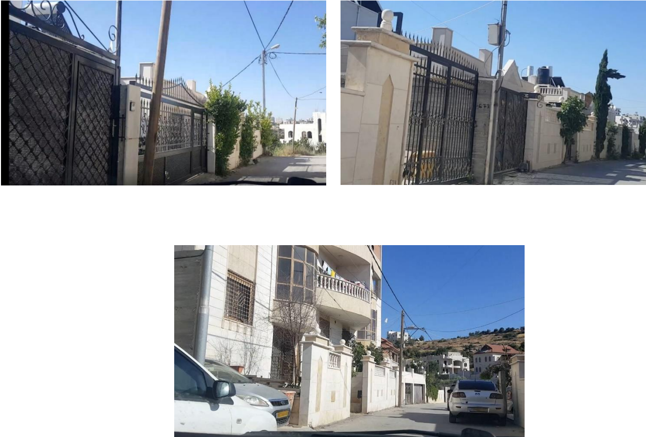
Figure 0.12: Photos of the gates in Al-Nejmeh residential complex.
