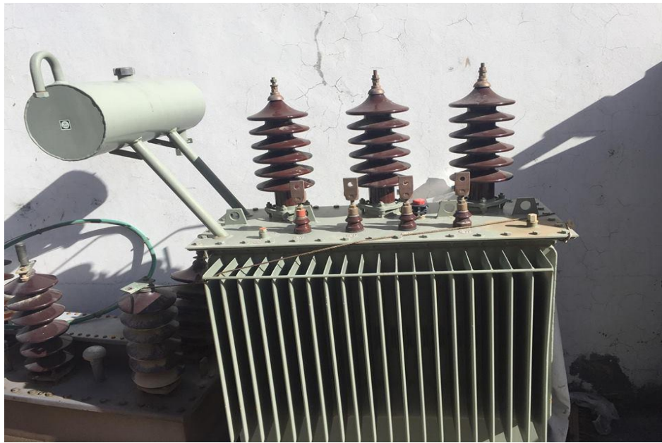
Figure2.6: Three-phase transformer
