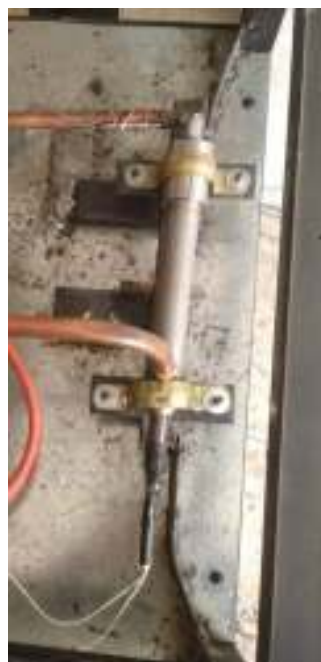
Figure 5.7: Heater after installation
