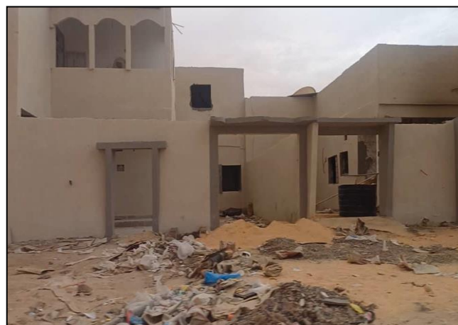
Figure 7. Maintenance operation of some damaged houses
