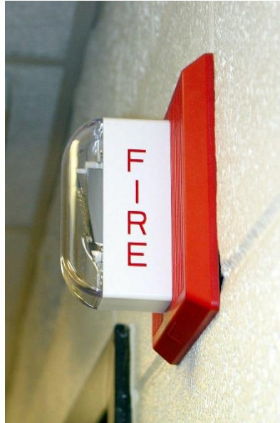
Figure 6.2 Visual alarm device
