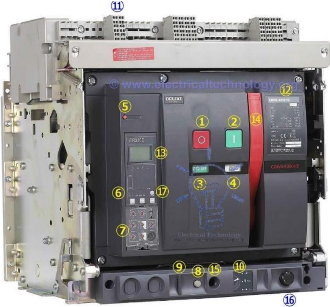
Figure 5.4 air circuit breaker [2]
