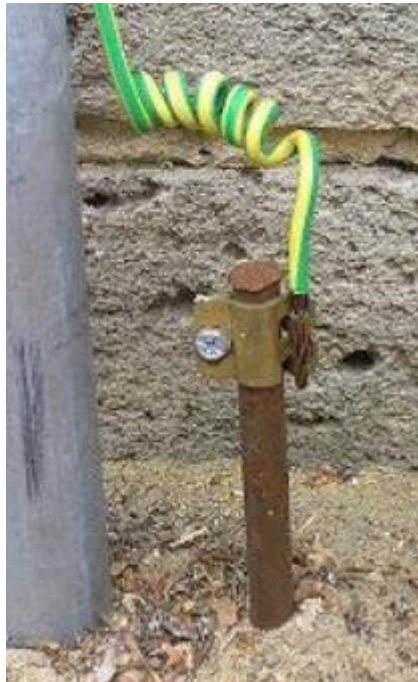
Figure 8.3 earthing electrodes [2]
