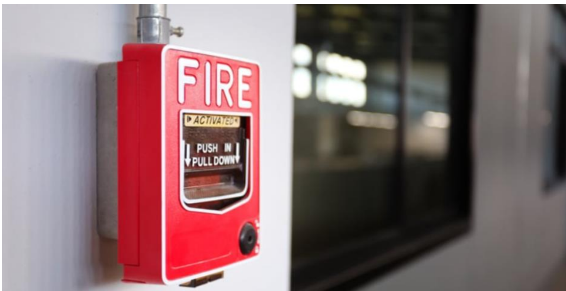
Figure 6.1 Manual Operating Units [10]
