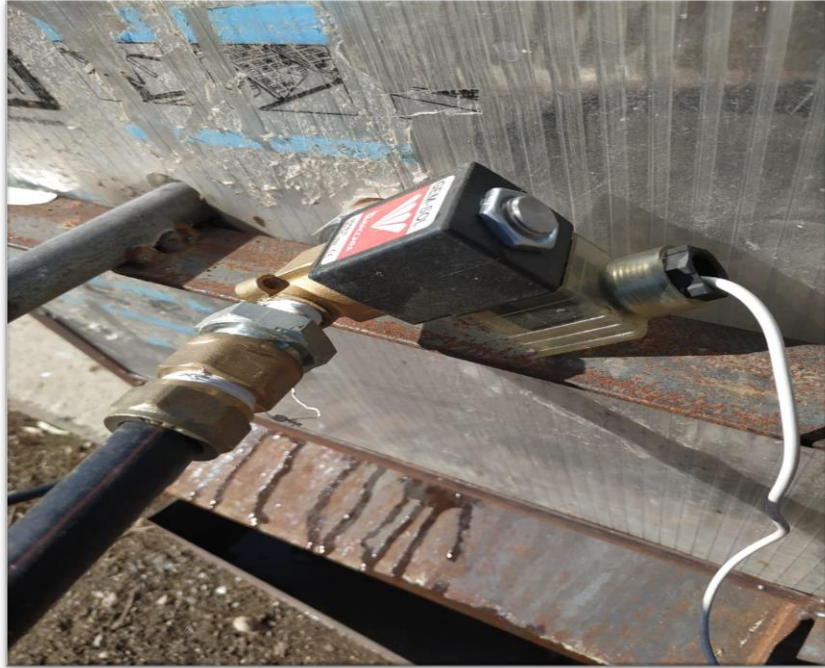
Figure 5.14: Solenoid valve
