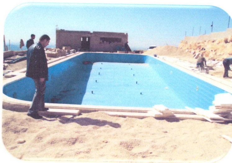
Figure (3.8): Construct floor inlets
