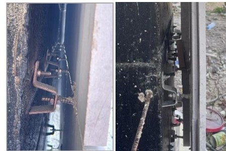
Figure 4-23: Installed bracket within the ventilated cavity, showing the waterproofed backing wall (Researcher, 2026)
