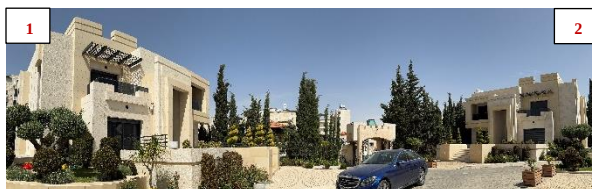
Figure 4-12 Panoramic view of the two buildings in Sha'abah (Researcher, 2026)
