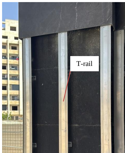
Figure 4-24: Vertical aluminium T-rails fixed to the waterproofed backing wall (Researcher, 2026)
