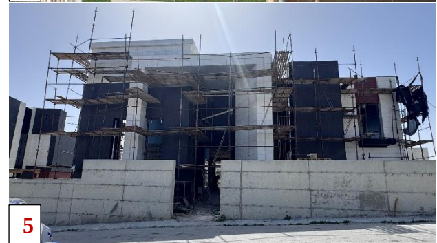
Figure 4-16 The mechanically fixed stone and porcelain-clad buildings 4 and 5, Farsh Al-Hawa, during the cladding phase (Researcher, 2026)
