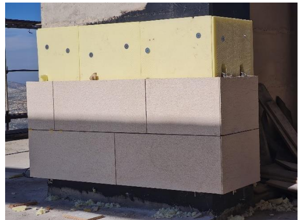
Figure 4-28: Construction stage of the external wall assembly in the case study buildings (Source: Mohammed Alamah, cladding contractor, 2010).
