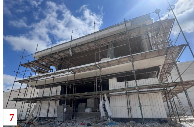
Figure 4-20: Building 7, Wadi Abu-Ektelah, during the cladding phase, showing the mechanically fixed stone cladding in progress (Researcher, 2026)
