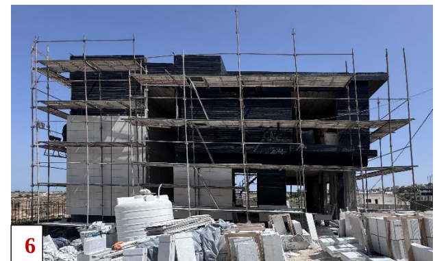
Figure 4-18: Building 6, Farsh Al-Hawa, during cladding installation, showing the bituminous waterproofing membrane on the structural wall and the partially completed mechanically fixed stone cladding (Researcher, 2026)
