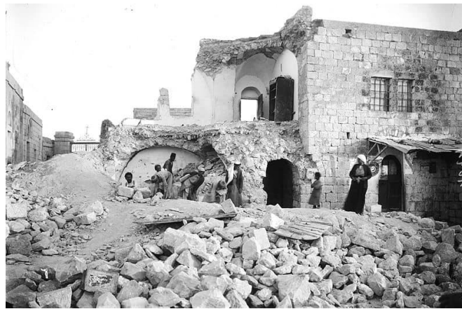
Figure 1.4: damage of the old buildings in Nablus.
