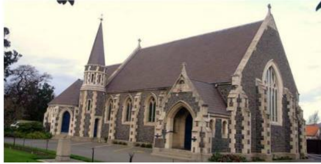
Figure 2.18: general view of St. James church. [26] (Araújo, Lourenço, Oliveira and Leite, 2012)
