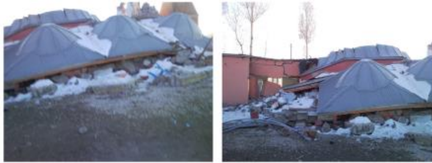
Figure 2.1: Collapsed masonry mosques with their dome.
