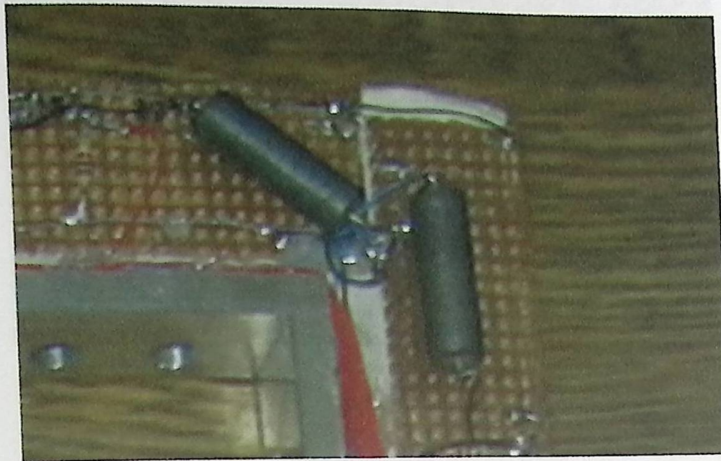
Figure 6.2: High Power Resistors
