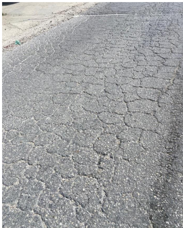
Figure 3.3: An image showing alligator cracks
