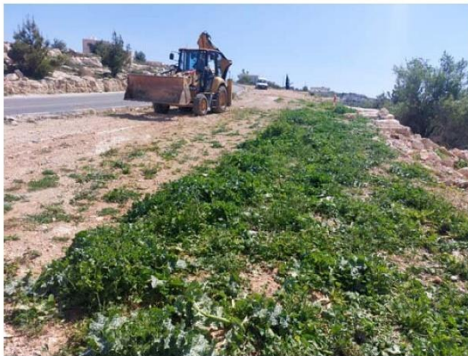
Photo -6- Photos (5 & 6) Site Condition
