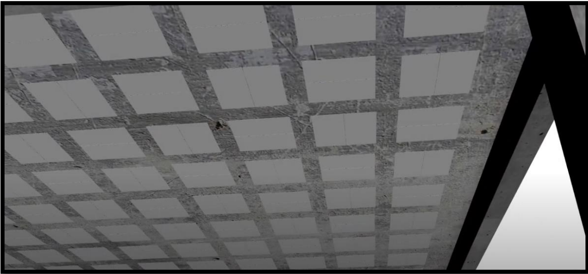
Figure 3-3:Two-way ribbed slab
