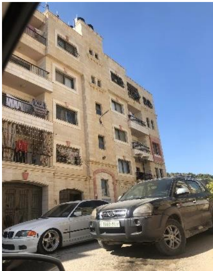
Figure 4-17: area (1) in King Abdullah Ben Abdul-Aziz residential complex showed parked cars and concrete structures (Source from researcher)
