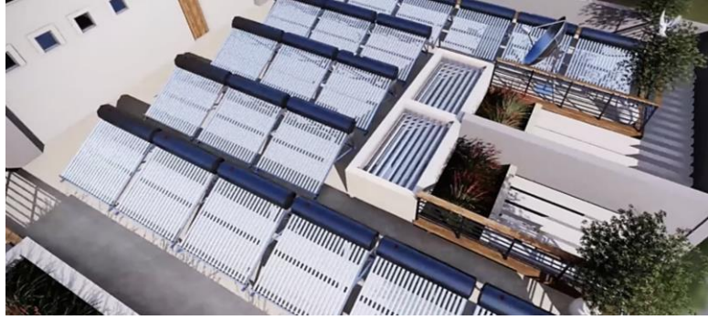
Fig. 4. 6: photovoltaic panels on the building's roof (SHTAYYA, 2018)
