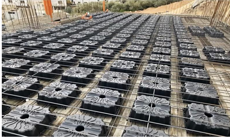
Fig. 4. 10: U-Boot Voided Slab System (SHTAYYA, 2018)
