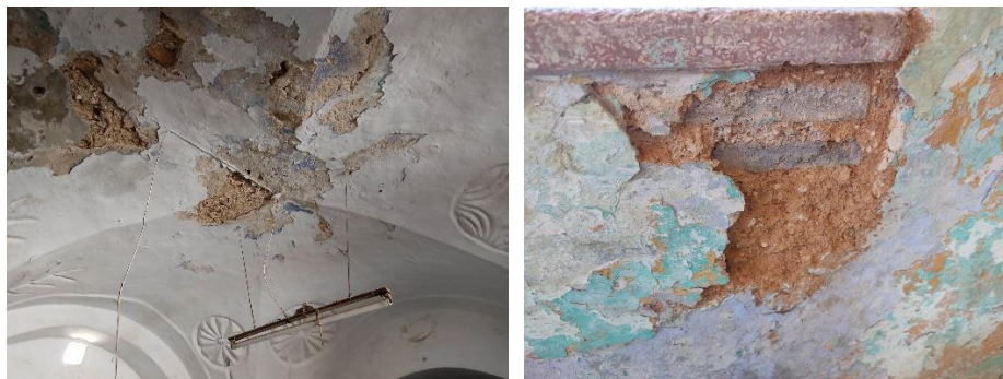
Figure 3.9: removal of lime mortar. Source: researcher
