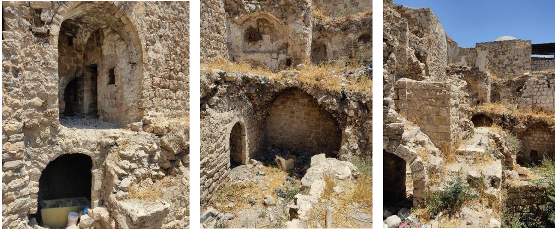
Figure 4.1: source location of historical stone from collaps building. Source: researcher
