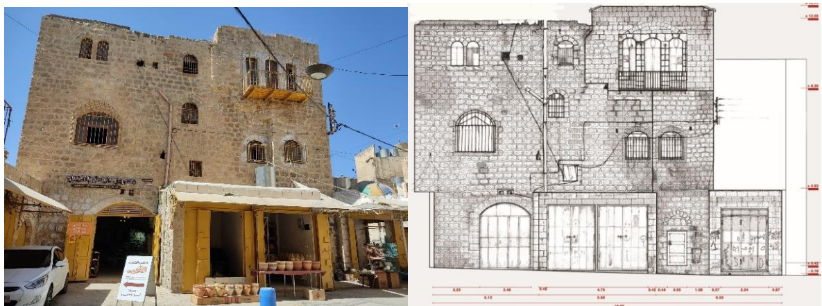
Figure3.3: Front facade of the building. Source: researcher
