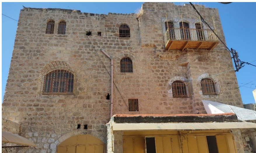
Figure 3.11: Good condition in external facades. Source: researcher
