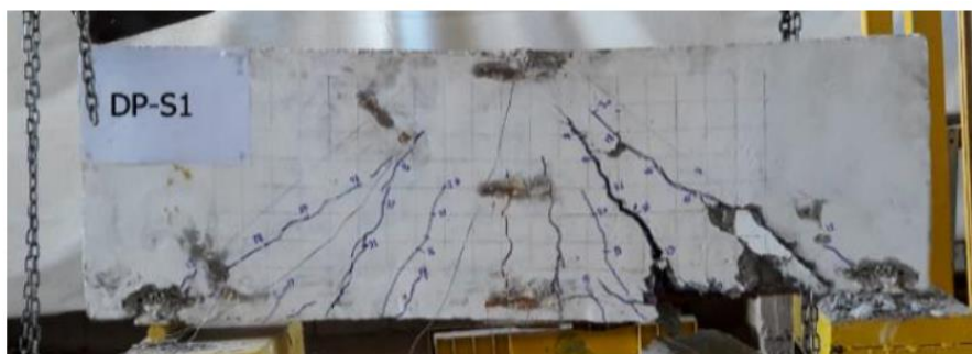
Figure 41 : Diagonal splitting failure of (DP-S1)
