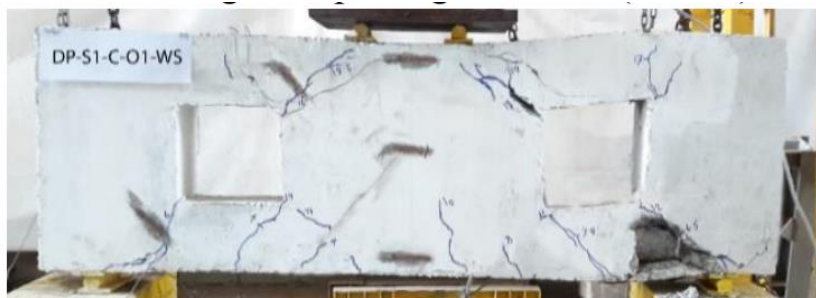
Figure 48 : Diagonal splitting failure of DP-S1-C-O1 Expermintal
