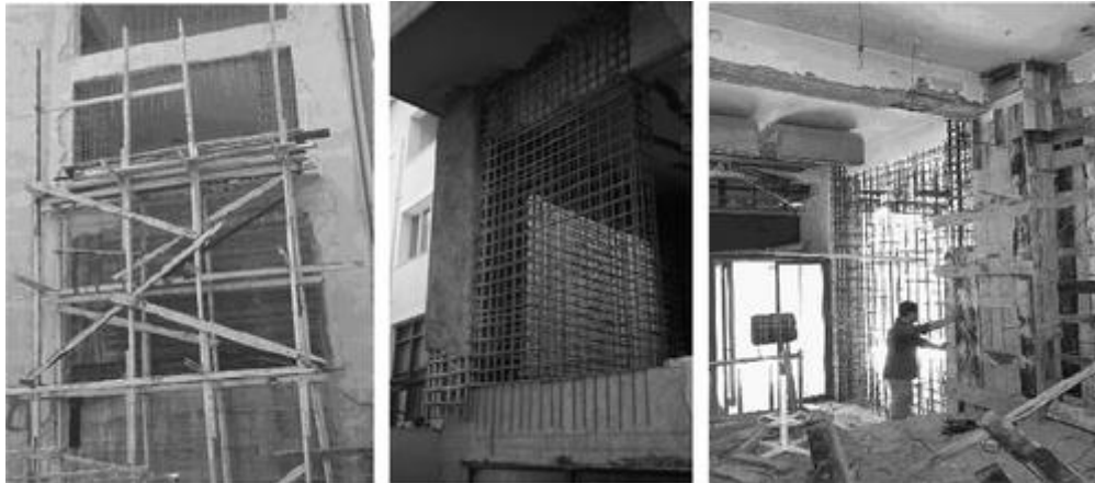
Figure 48 - Cast-in-place infill walls
