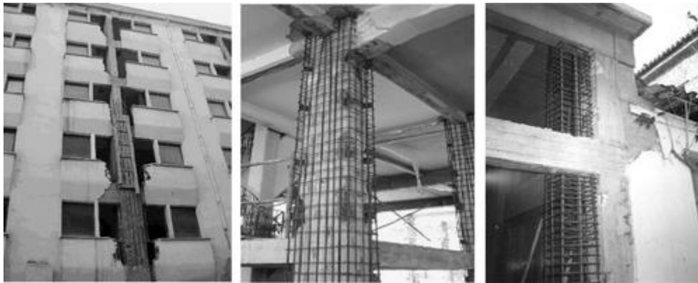
Figure 47 - Reinforced concrete jacketing technique
