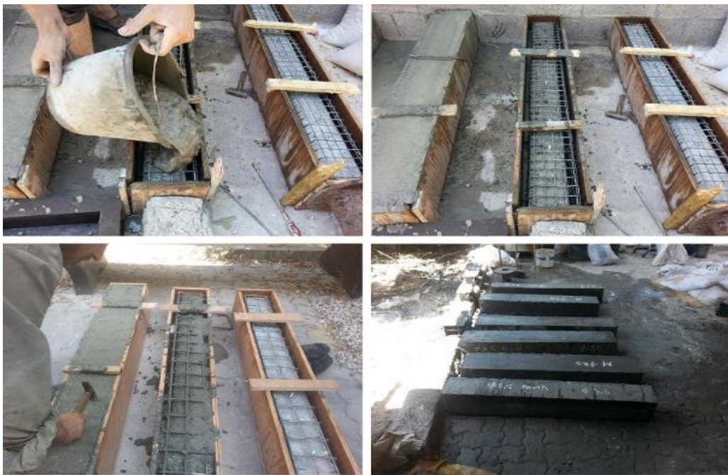
Figure 23 SCC pouring process.
