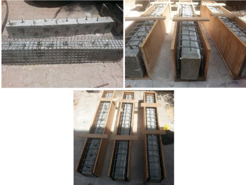
Figure 22 Preparation of the wooden moulds.
