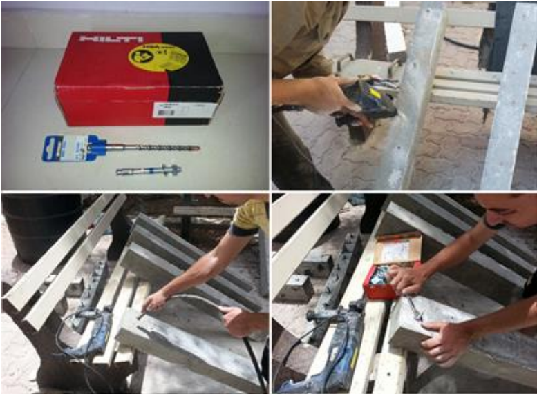
Figure 19 Hilti type shear connectors installation.
