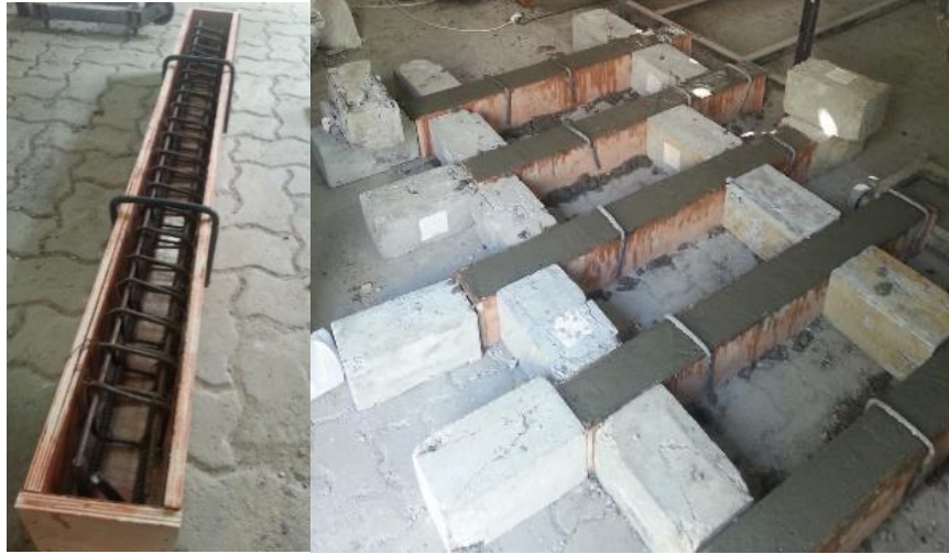
Figure 21 Production of the initial core beams.
