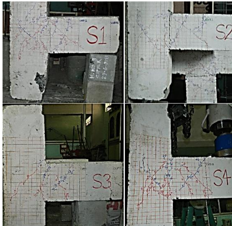
Figure 30 The experimental crack pattern.
