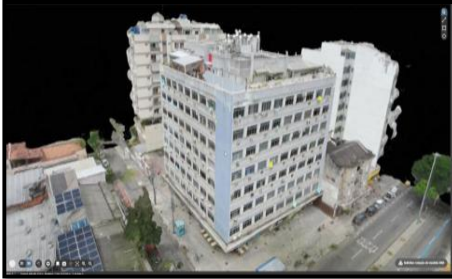
Figure 2-4.5 Multi-storey building inspections
