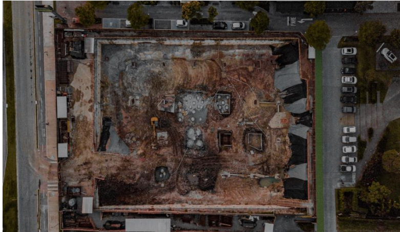
Figure 2-2.7 Using Drones in Construction site monitoring and manegment
