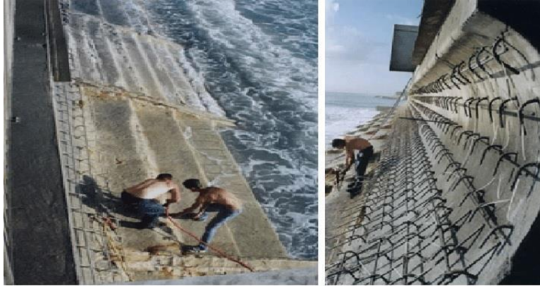
Figure 13 Seawall restoration in Palm Beach Florida, USA (Aslan FRP, 2018)
