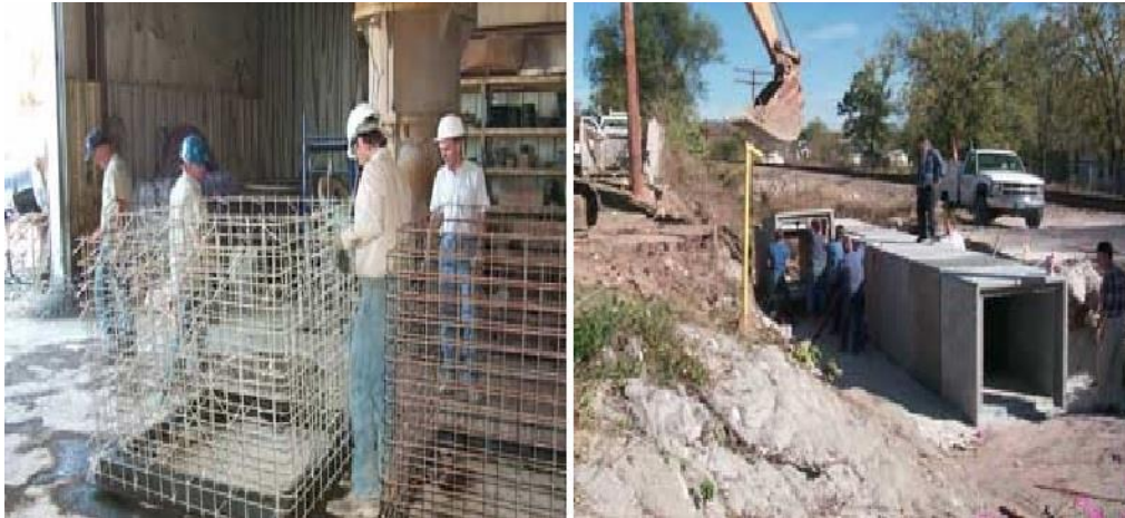
Figure 17 Culvert bridge in City of Rolla, Phelps County, Missouri (Nanni, 2000)
