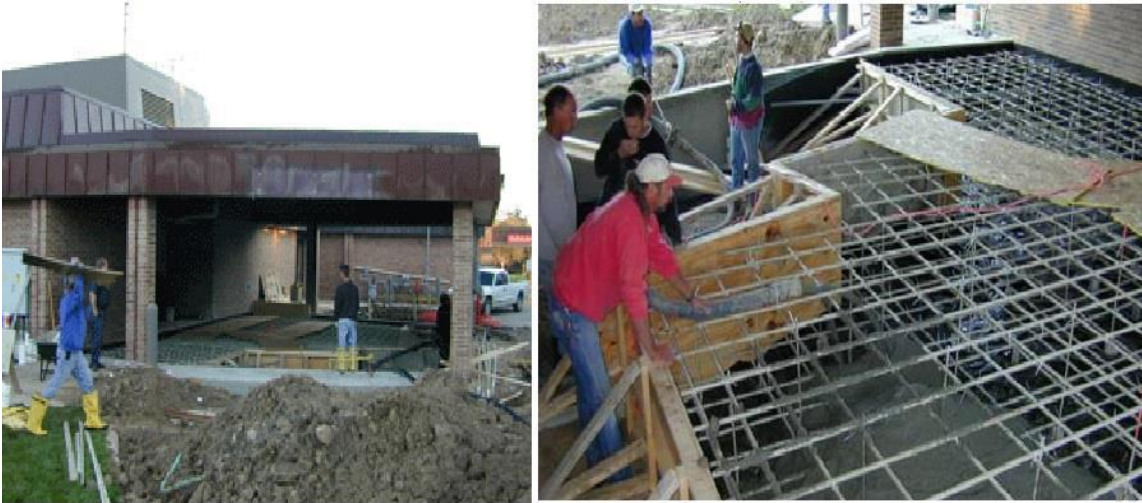
Figure 12 Trauma Centre in York Hospital (Aslan FRP, 2022b).
