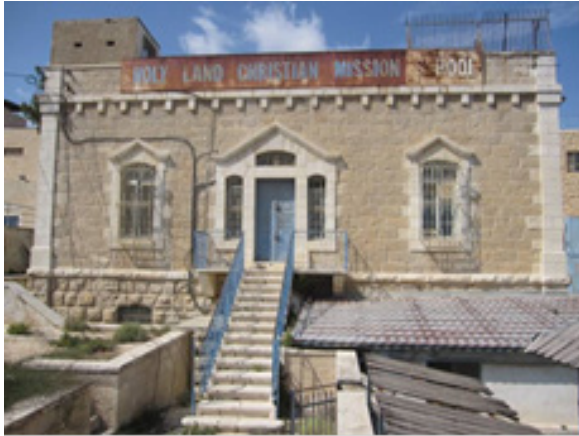
Figure 1. General view of the building –North West Facades
