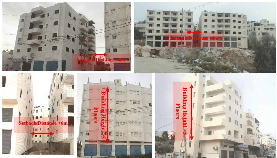
Figure 4.2: Multi-story residential buildings in residential B-Zone.
