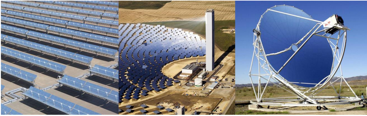
Figure (2.1) From Left to right, Parabolic, Tower, Dish Stirling
