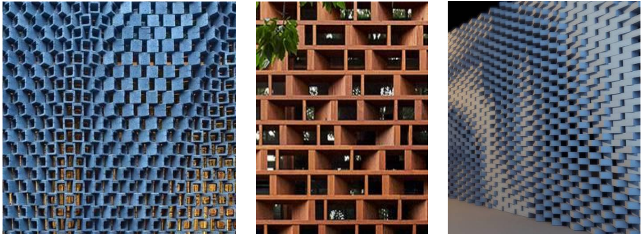
Figure 5.8: Illustrative examples of changing rotational angles of the envelope's perforated layer. References (left to right), < https://it.pinterest.com/pin/426223552216021729/ >, < http://www.archdaily.com/620039/local-house-make-architecture >, < http://4.bp.blogspot.com/-vA7kzOokaCY/UYYUcqzBMnI/AAAAAAAAAPo/9pTxPwEoluw/s640/Render+3.0127.jpg >, (09/2016).
