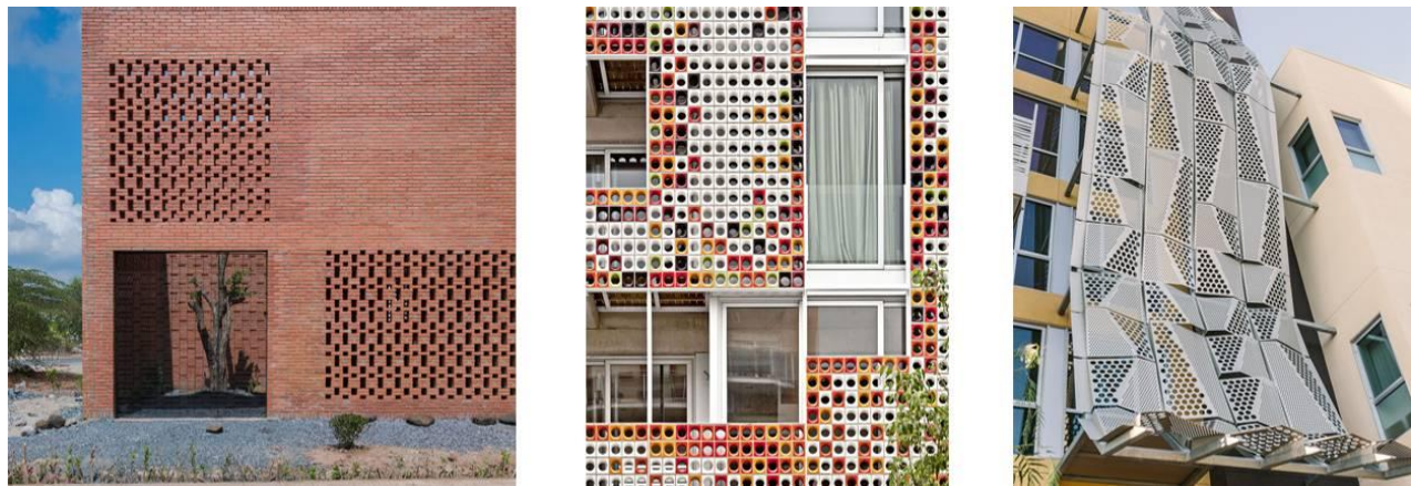
Figure 4.9: Changing perforation's configuration in different cases, references from left to right: < http://www.archdaily.com/789533/lt-house-tropical-space >, < http://www.contemporist.com/2015/03/02/a-facade-of-colorful-ceramic-blocks-cover-this-apartment-building/ >, < http://amicoglobal.com/fabricated-products/applications/facades-sunscreens/ >, all accessed on (05/2016).
