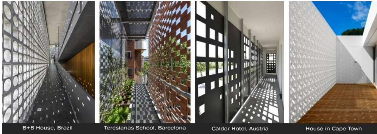
Figure 4.7: Examples of accessible air cavity in different cases of perforated envelopes (Germanà et. al., 2015).
