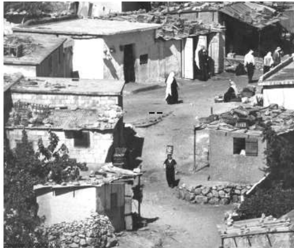
Figure (4.3): Dheisheh first concrete block houses. Source: UNRWA, 2008.
