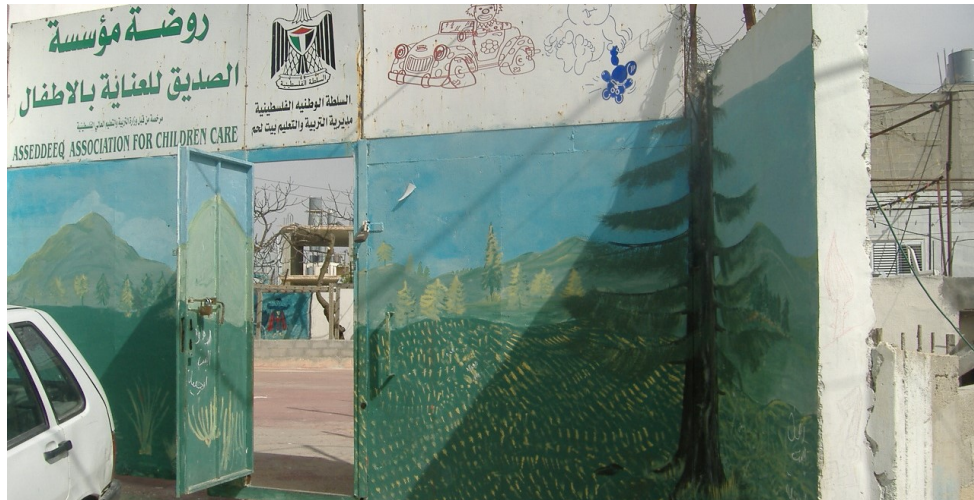
Figure (6.14): Kindergarten external walls. 1
