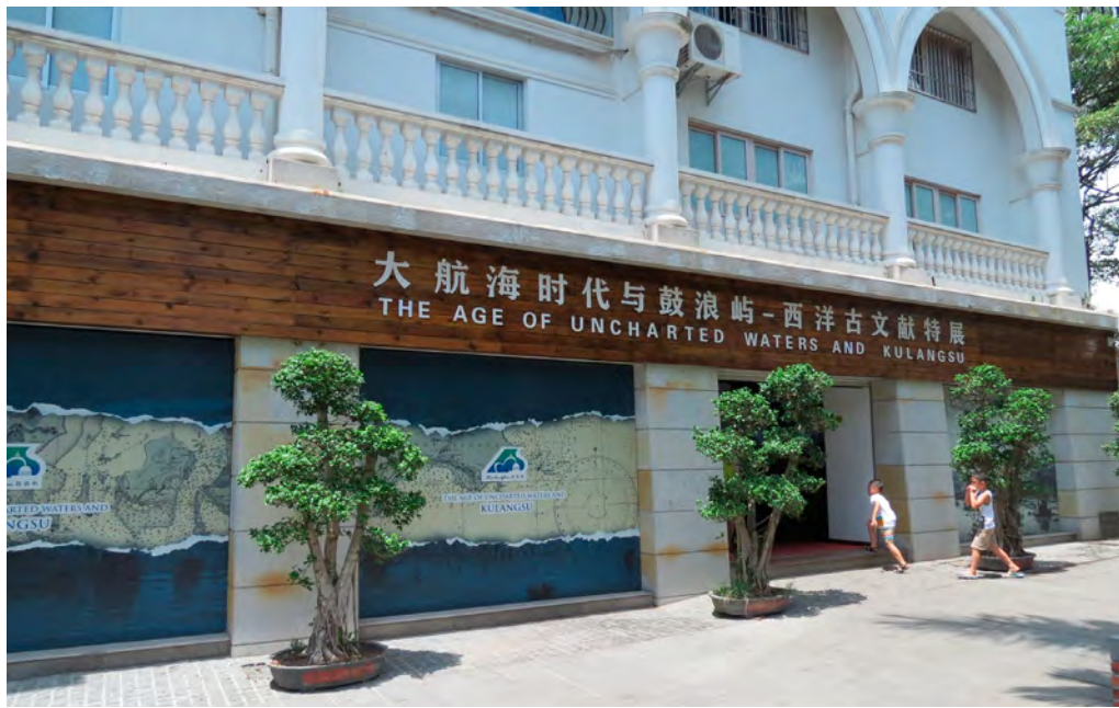
Figure 3: frontal image of 'The Age of uncharted waters and Kulangsu' museum, taken by Law, 2014.
