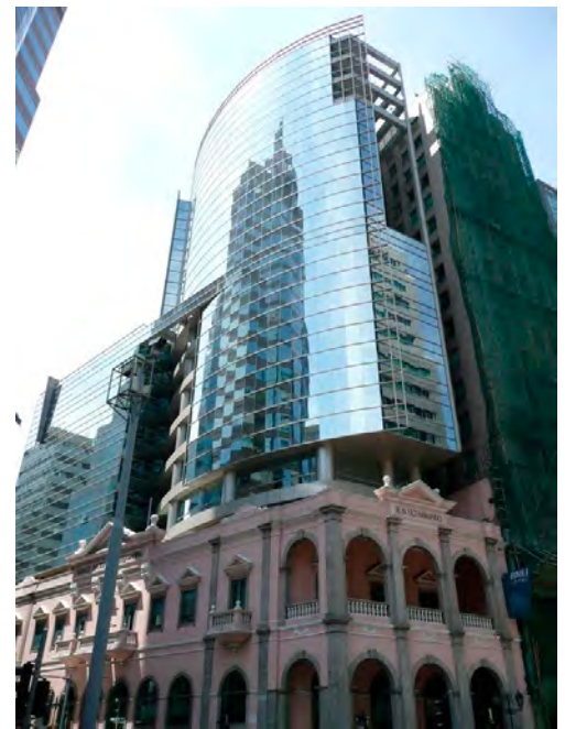
Figure 1: Banco Nacional Ultramarino building in Macau (picture taken on 19 June 2007 by Hinto under CC BY 2.5)
