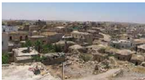
Figure 3- A general view of the old town of Al-Dahiriya Village (By RIWAQ)
