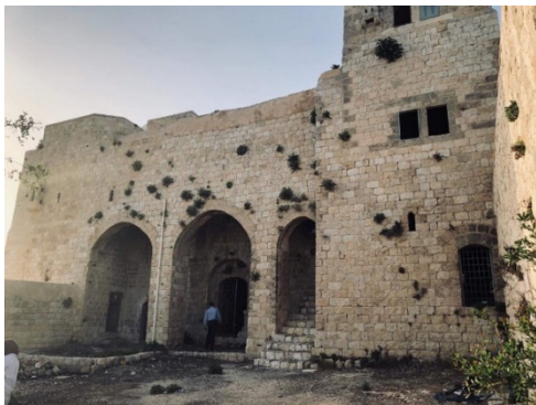
Figure 8: Al Hakem palace main entrance, Kour, Tulkarm.
