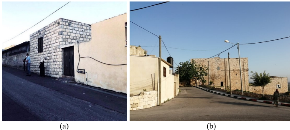
Figure 10: Plastered concrete block additions to buildings, Kour. (Source: Researcher, 2019.)
