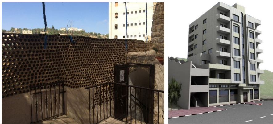
Figure 14. Comparison at the level of the openings, the use of “Kizan” for privacy and cooling purposes, Old (Left); outdoor areas, such as balconies, without visual privacy, New (f).
