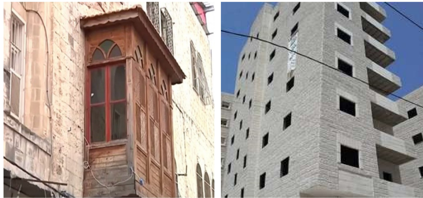
Figure 11. Comparison at the level of the openings, use of shading and privacy elements as the “Mashrabiya,” Old (Left); non-shaded openings, New (Right).
