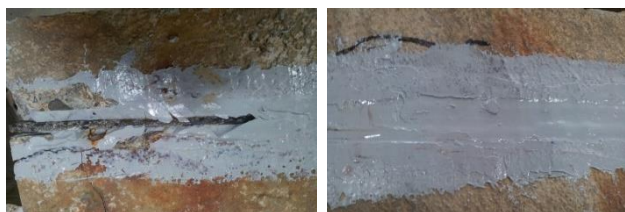
a. Before Re-repairing. b. After Re-Repairing.
