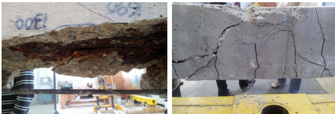
a) A1CL3-R Corroded
