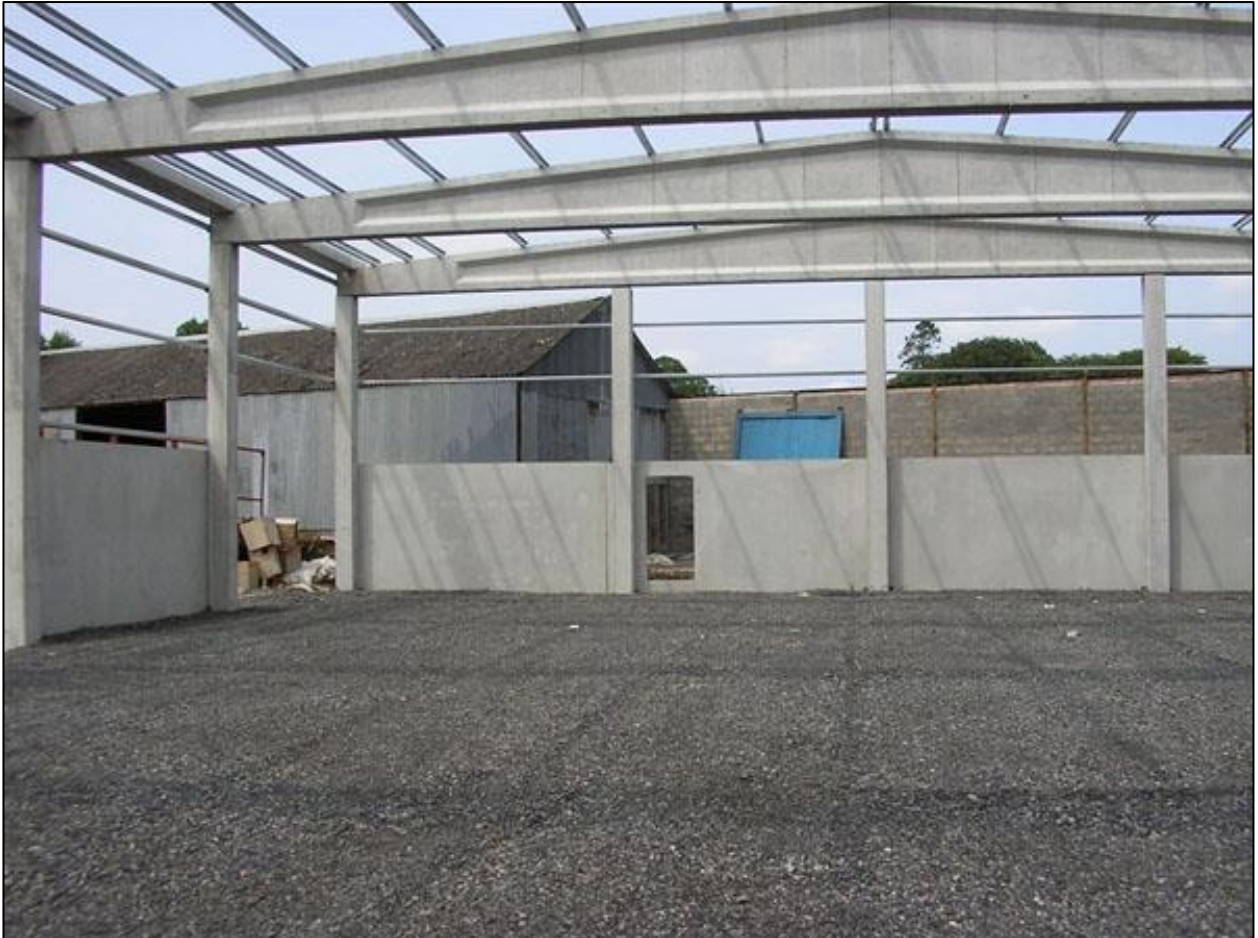
Figure (3-13): Frame Structure.
