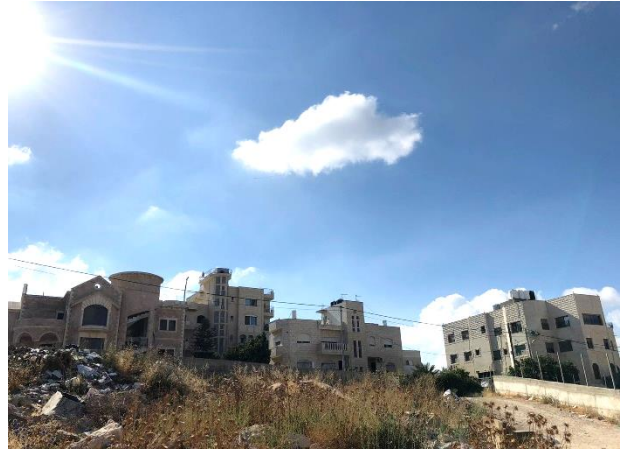
figure 2. 15: northern west view – entrance from street
