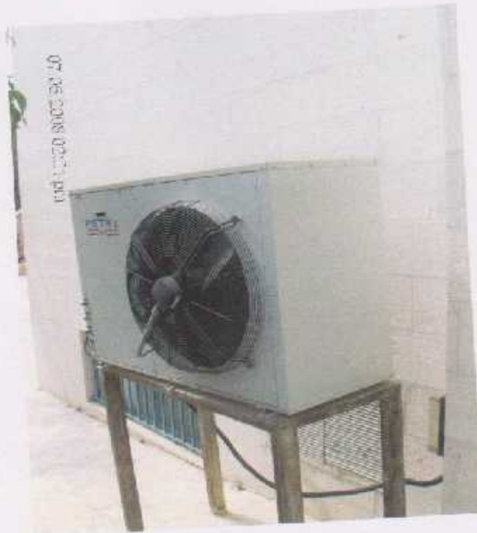
Figure 2.4: Ducted Split Unit (DSP)-(outdoor unit)
