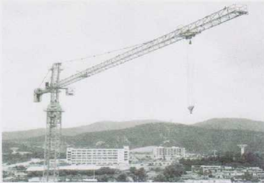
Figure (1.4): Tower Crane.
