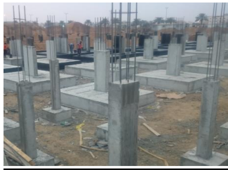
Figure(3- 7): Isolated Footing
