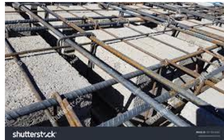
Figure(3- 4):Two way ribbed slab
