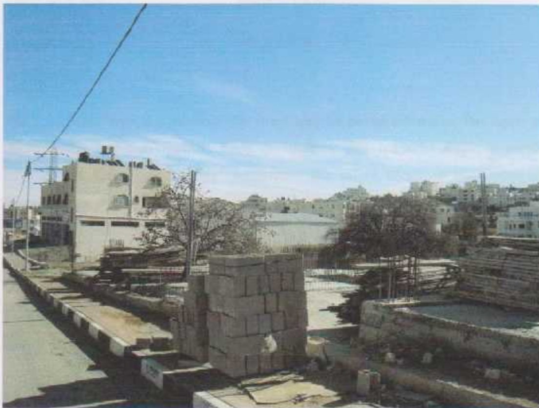
Figure 6-2: constructions hardware on sidewalks Source: researchers lens
