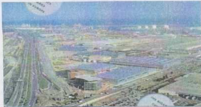
Figure 3-21 : Parc Logistic under construction Source: Annual report of El Consorci
