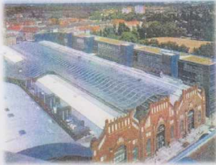
Figure 3-14 : after revitalization Source : http://www.am-borsigturm.de/
