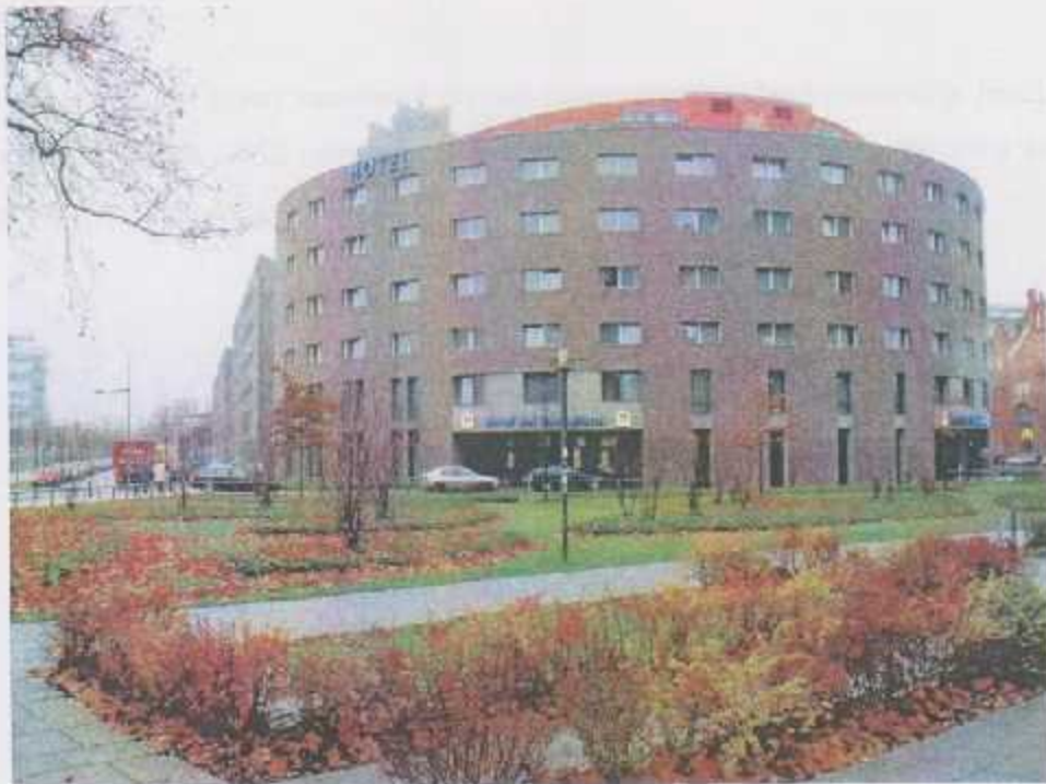
Figure 3-16 : view of the hotel
