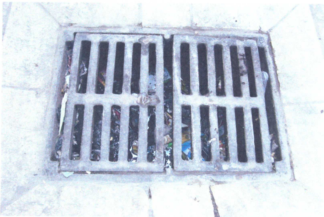
Fig 3.17 the system inlets in the Old City
