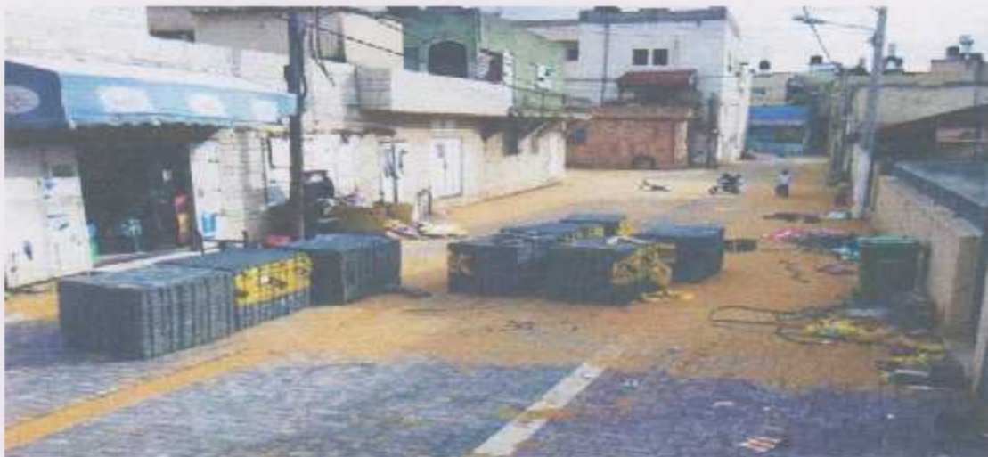
Figure 3.8. The roads in the Old City [ 3 ]
